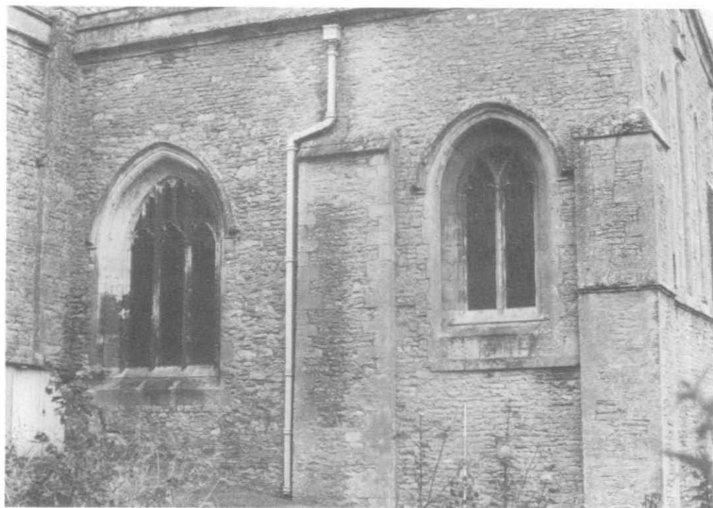
Plate 1. The external south wall of the chancel, showing the Romanesque walling and buttress ( centre ) abutted by the 13th-century eastwards extension with its string-course ( right ).
